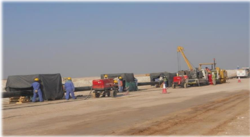
U/G 10" PIPELINE CONSTRUCTION - 49 KM - CCED
