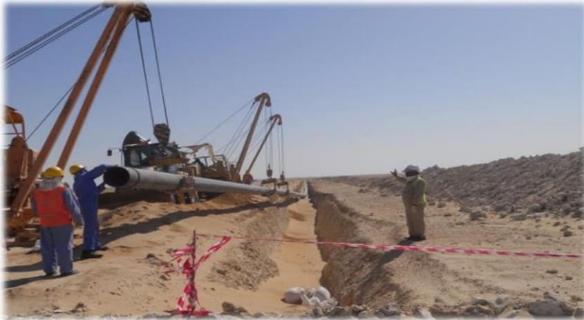
U/G 16" PIPELINE CONSTRUCTION – 72 KM - CCED
