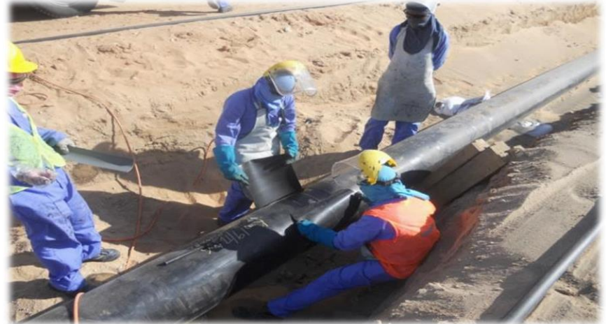
U/G 16" PIPELINE CONSTRUCTION – 72 KM - CCED
