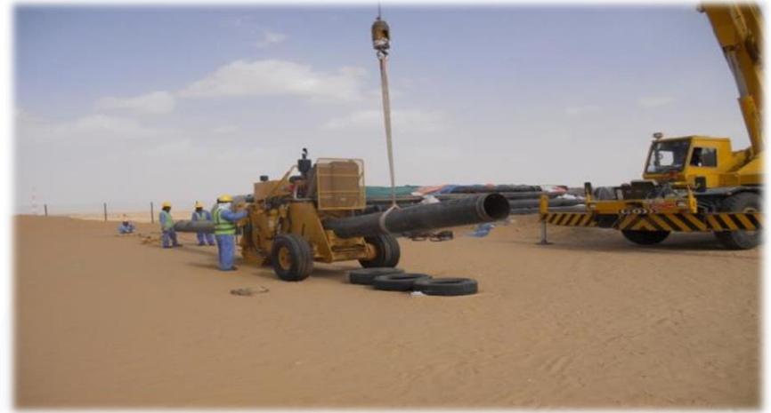
U/G 10" PIPELINE CONSTRUCTION - 49 KM - CCED
